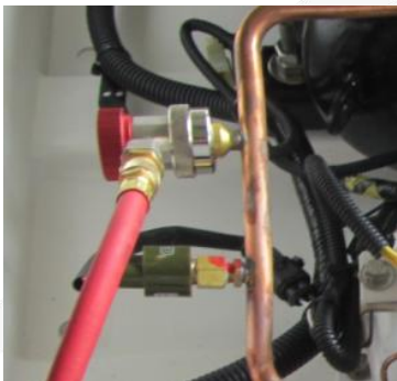
Connect yellow hose to vacuum pump Connect blue hose to low pressure value Connect the red hose to high pressure value
