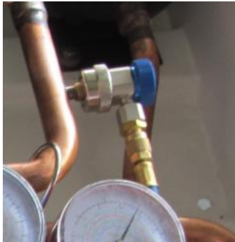
Connect yellow hose to vacuum pump Connect blue hose to low pressure value Connect the red hose to high pressure value
